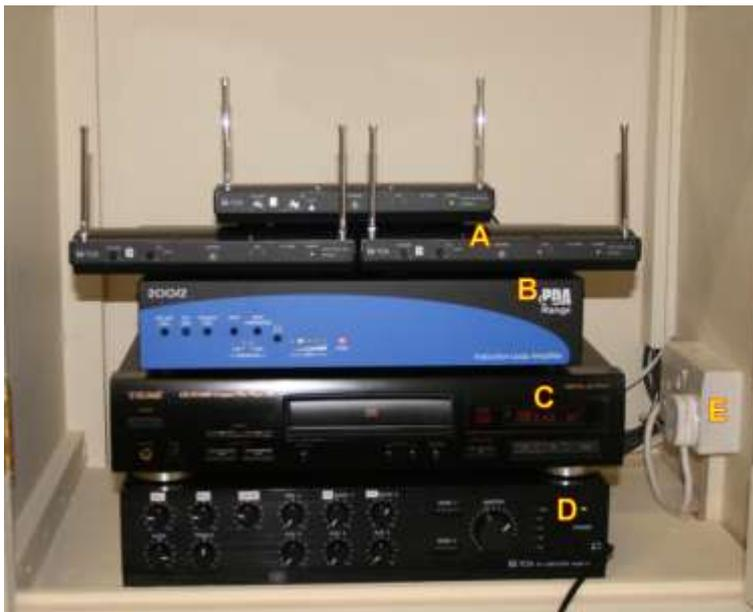
**When using this equipment switch on power from the socket in the Equipment cupboard (power point furthest from the door of the cupboard). Then press the 'POWER' button on unit 'D', and the CD Player above (C), which will illuminate immediately. The Microphone equipment and the Loop system automatically become activated.**
